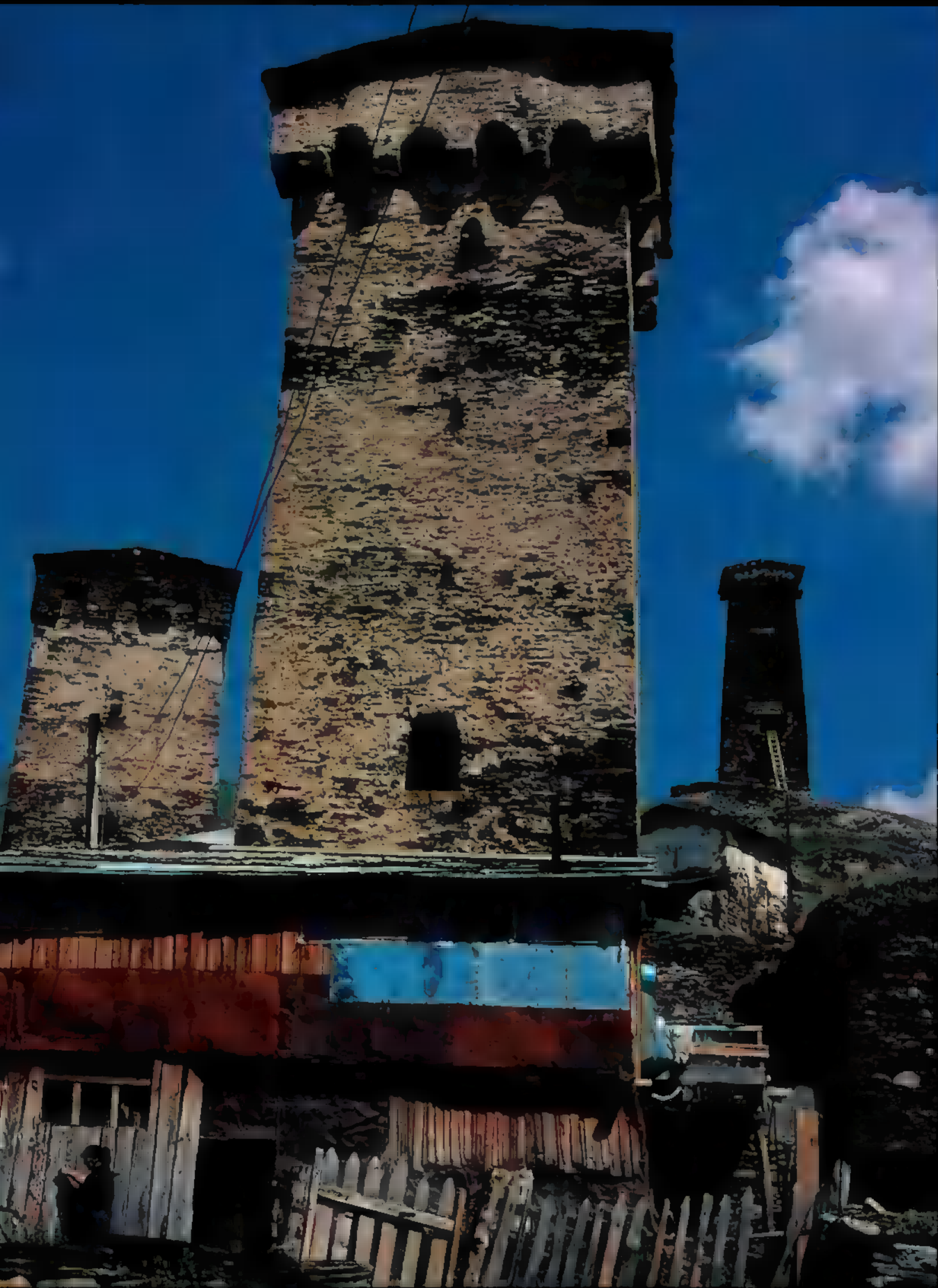
medieval towers of the village settlement in the high mountains of Georgia. Although still ruled by clans, the village cannot escape the eternal cross fire from the world below.
